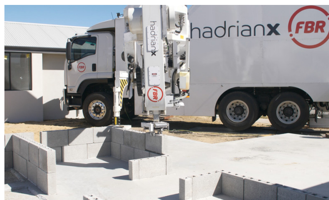
Hadrian X bricklaying robot. PHOTO | COURTESY
